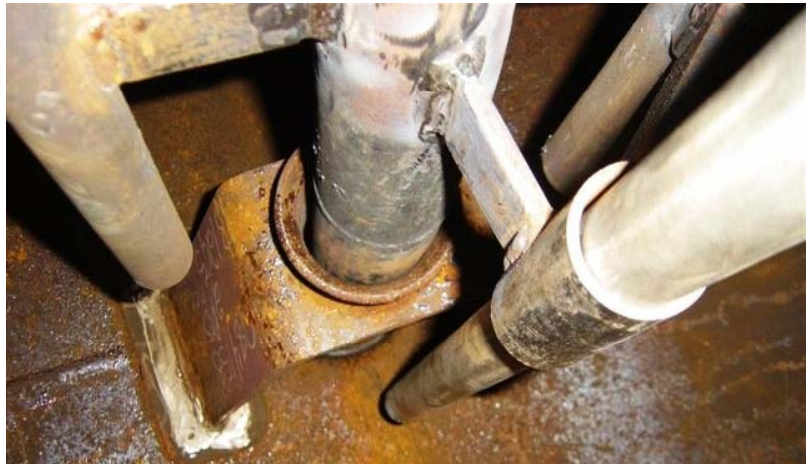
BEFORE: Example of a Conventional Tank Car (Welded) Eduction Pipe set-up.
